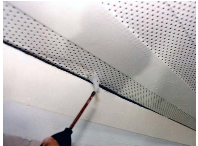
Figure 5. A smoke pencil test shows how air is drawn into a perforated metal ceiling panel.
